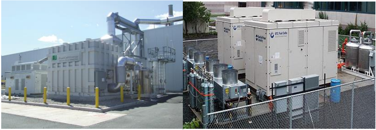
Figure 8: On left: fuel cell used in power plants; on right: fuel cell used on a building.
